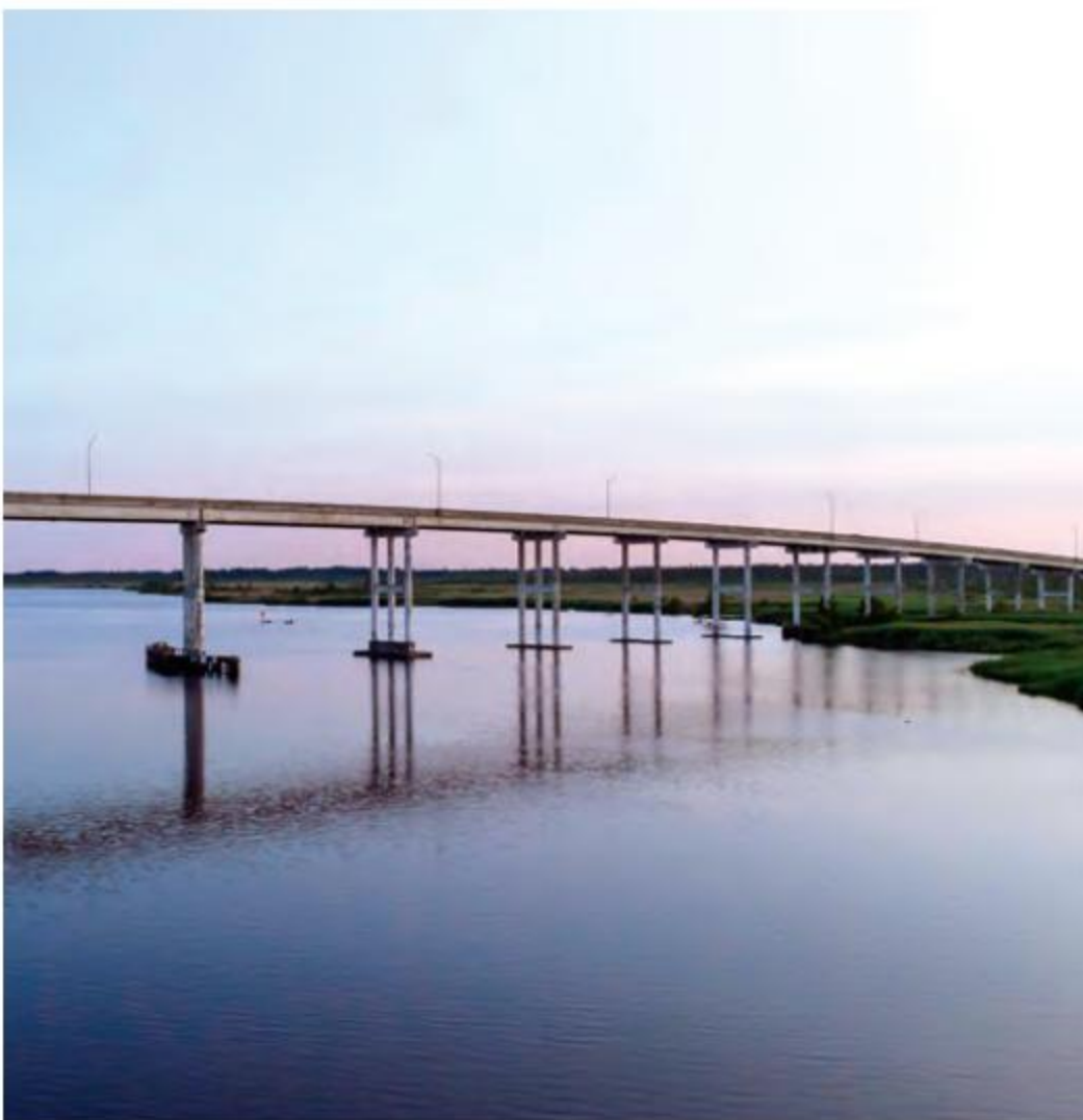
PUNGO FERRY BRIDGE
